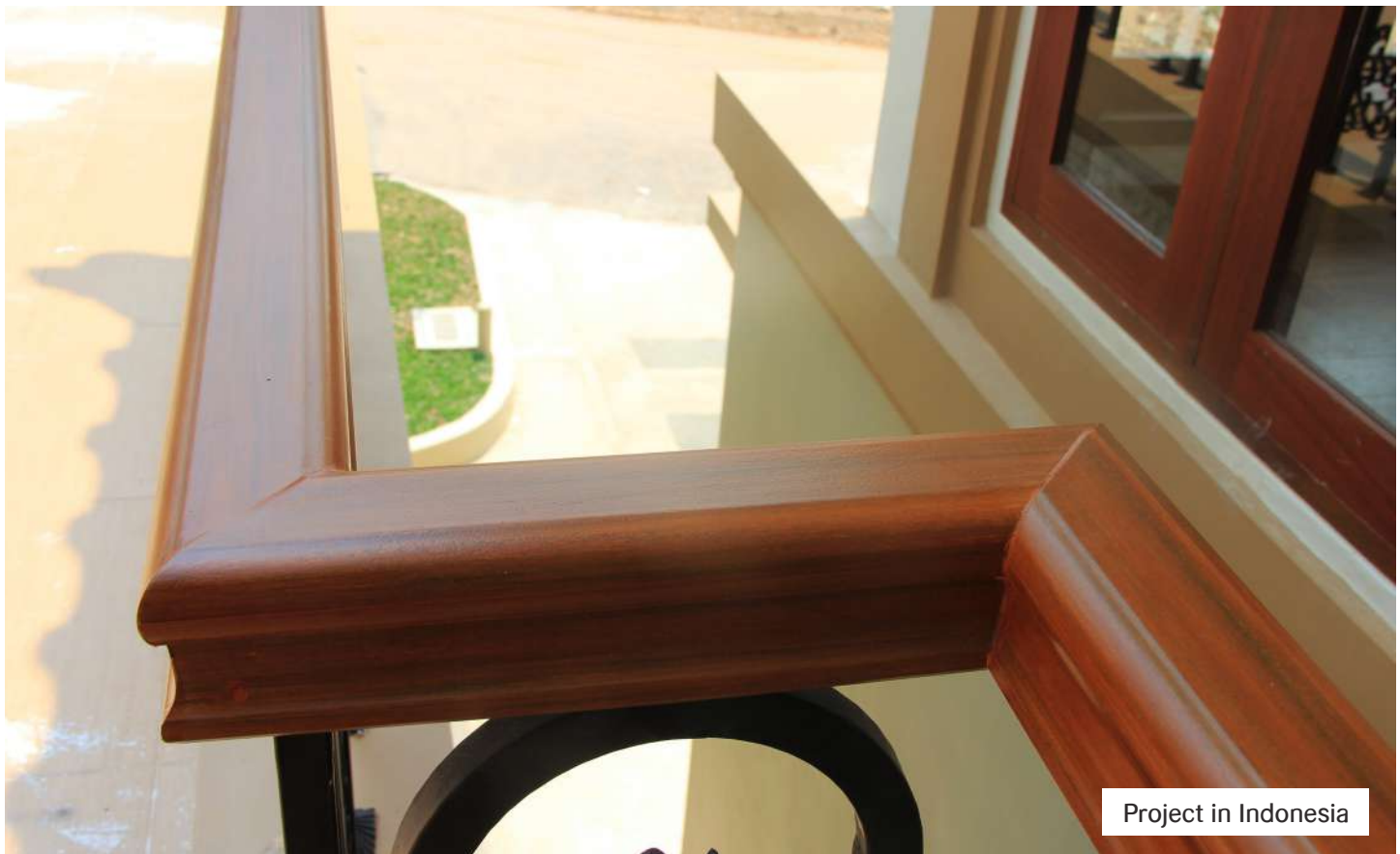
Project in Indonesia
